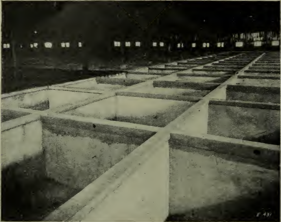
FIG. 2. CONCRETE TANKS FOR TANNING LIQUORS.
